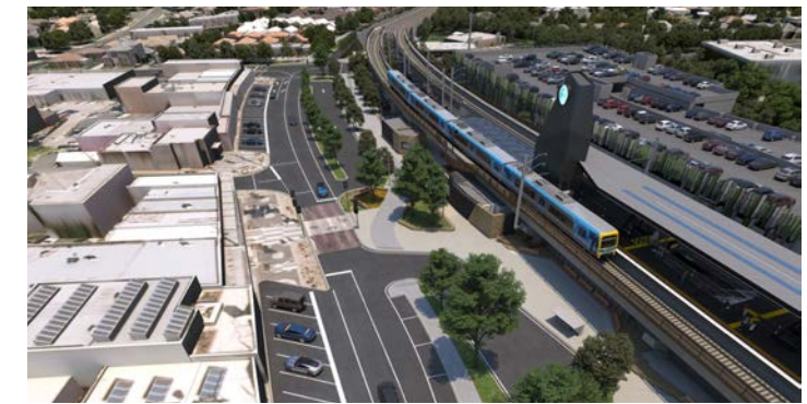
Mooroolbark level crossing and station. Source: LXRP
