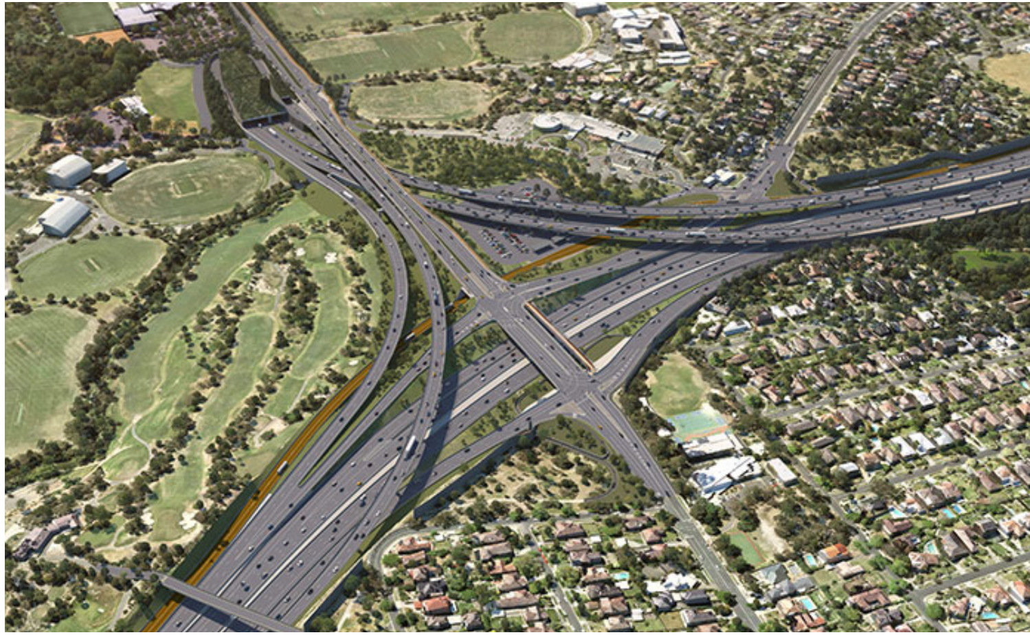
The southern connector of the North East Link project at the Eastern Freeway Source: NEL Project
