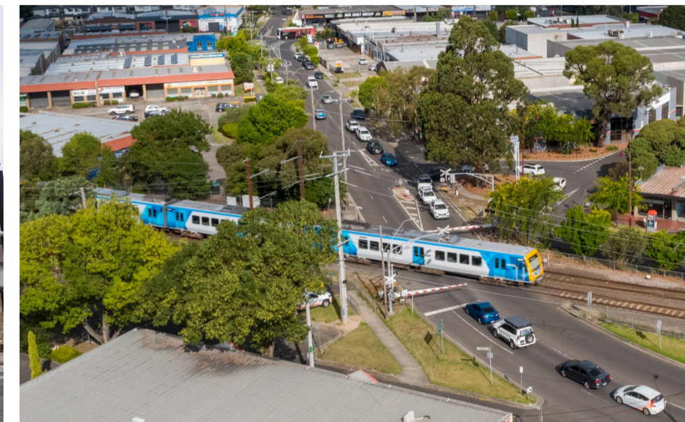
The Coolstore Road crossing is currently being prepared for removal.
