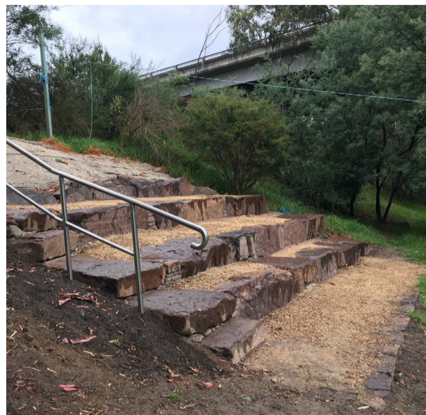
The new access point on the Yarra River in Templestowe.
